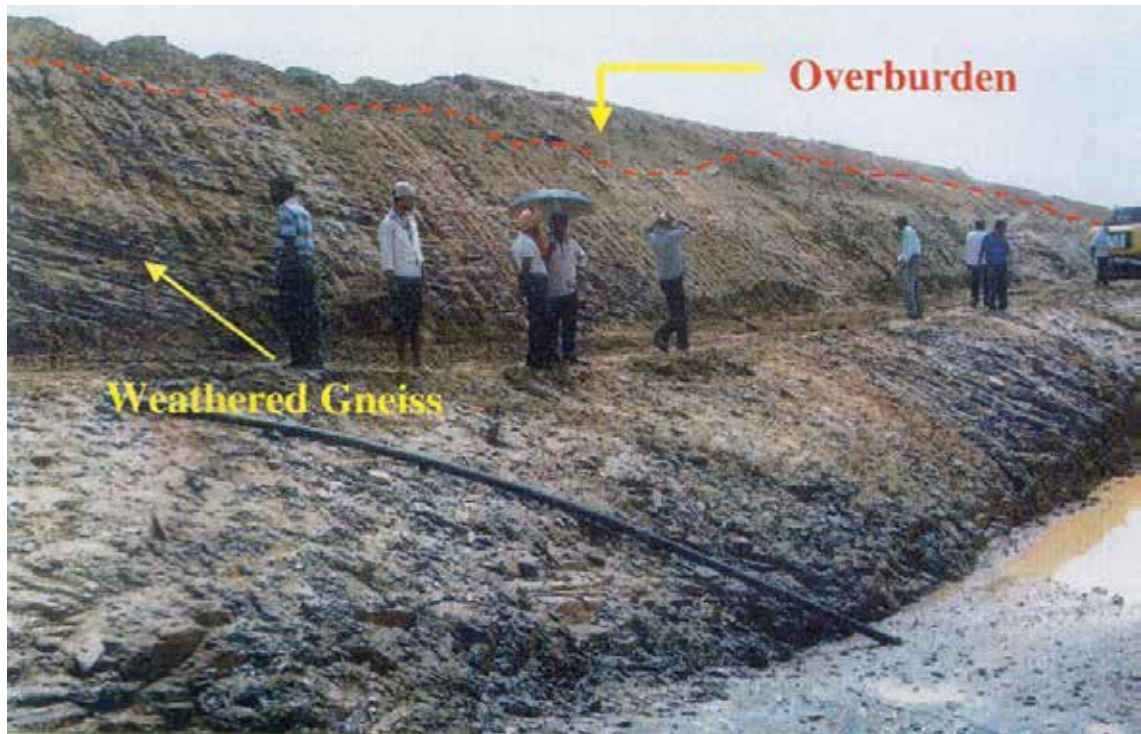
Picture 8 Upstream wall of parallel C-O-T showing weathered granite gneiss below soil overburden without sand layer at RD 1280m (Ch 42)
