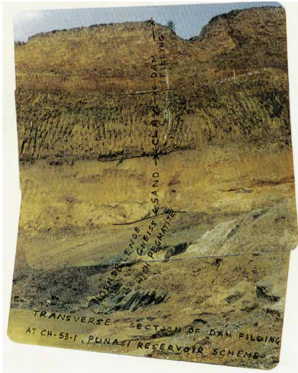
Picture 3 Vertical cross-sections at RD1616m (Ch 53) on the edge of the left bank showing sand layer underlain by rocky strata below dam filling.
