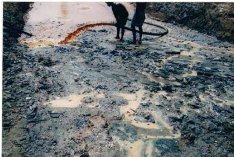
Picture 1 Hornblende gneiss rock at the cut-off trench bottom at RD 1951m (Ch 64) on right bank
