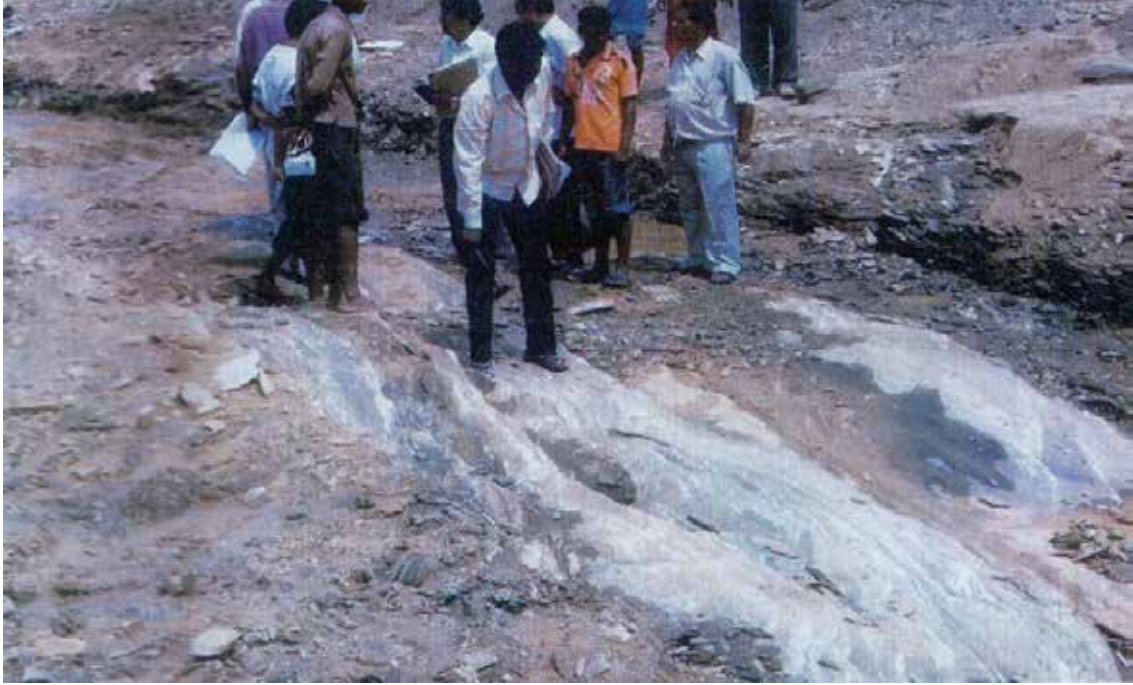
Picture 6 Fresh granite gneiss at C-O-T bed of parallel cut-off on left bank at RD 1265m (Ch 41.5)
